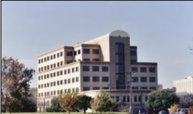
Brown-Heatly Building Offices of Texas Health & Human Services Commission
